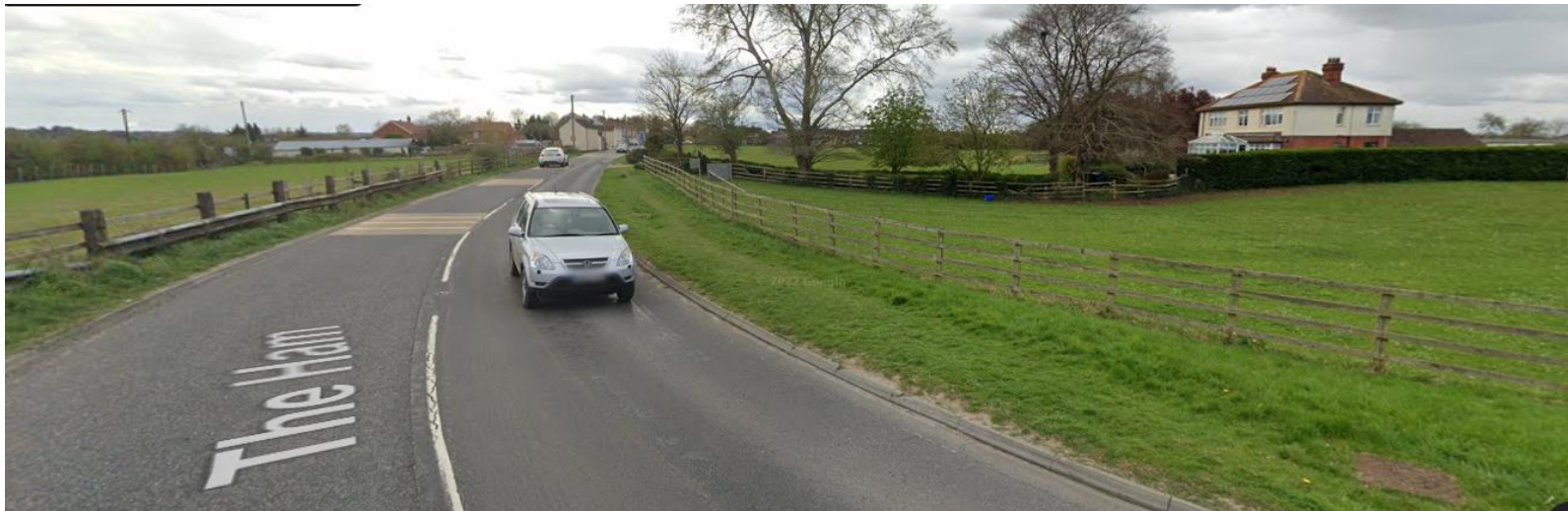
The junction of Hawkeridge Road and The Ham with the site on the right and Glenmore Farmhouse (to remain)
