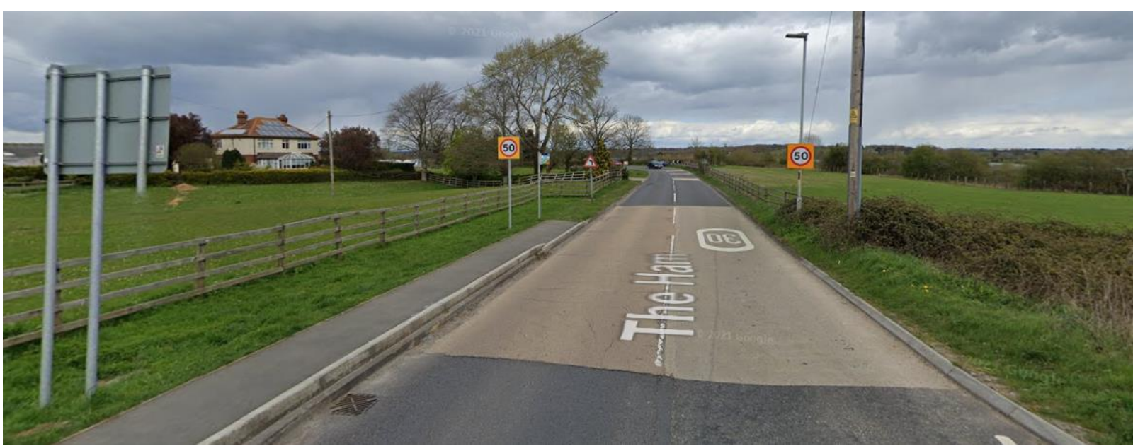
View along the Ham at the junction with Hawkeridge Road - where the proposed access will be
