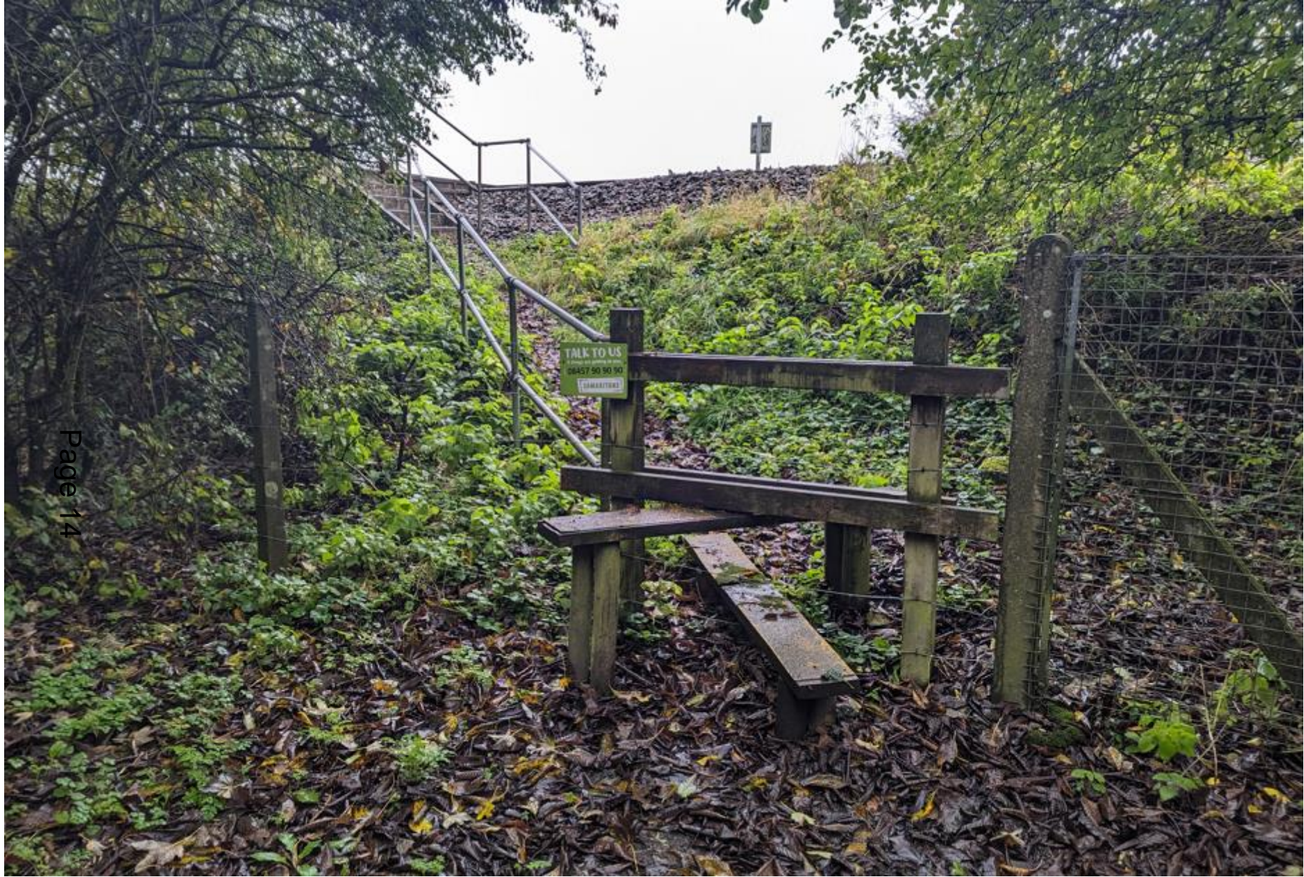
View of WARM18 level crossing (western side of railway)
