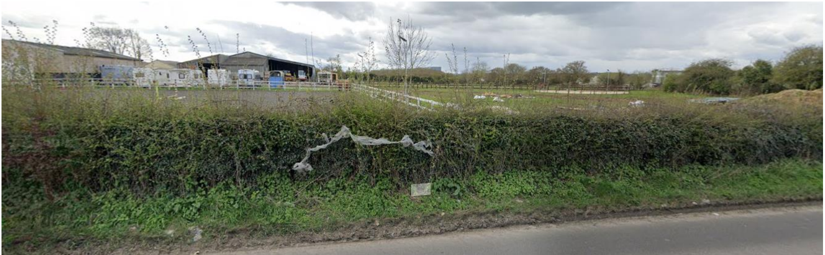
Looking towards the northeast edge of the site from Hawkeridge Road
